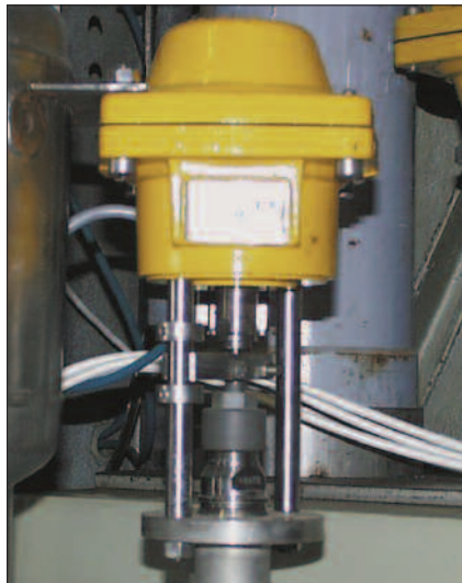
Model 2020 on a pilot plant - HF & Fluorine service - USA
